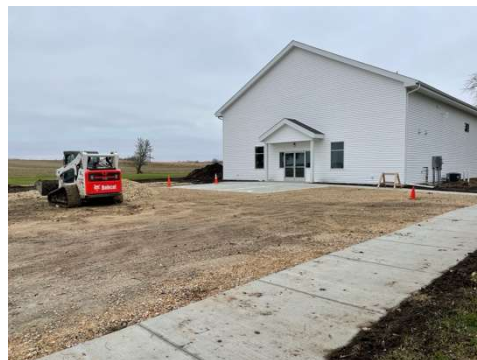
Gravel, handicap parking, and sidewalk installed.
